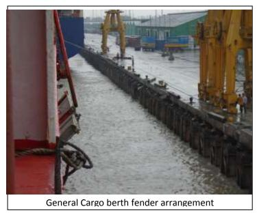
The timber claddings would also protect the ship's hull from the sharp upper edge of the 'I' beams as vessels would move up and down with tide or during loading and unloading.
