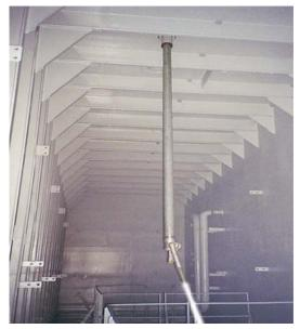
Tank Cleaning machine in operation.
